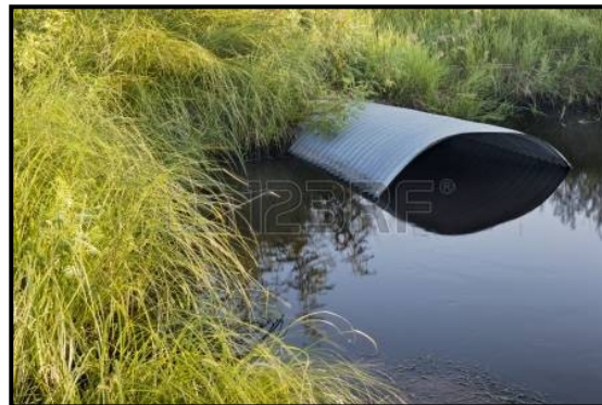
Undersized culvert
